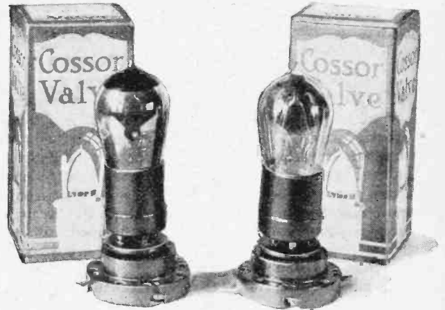
Valves of the new Coszor "Point One" class. The H.F. valve (red top) and Detector valve (plain top).
